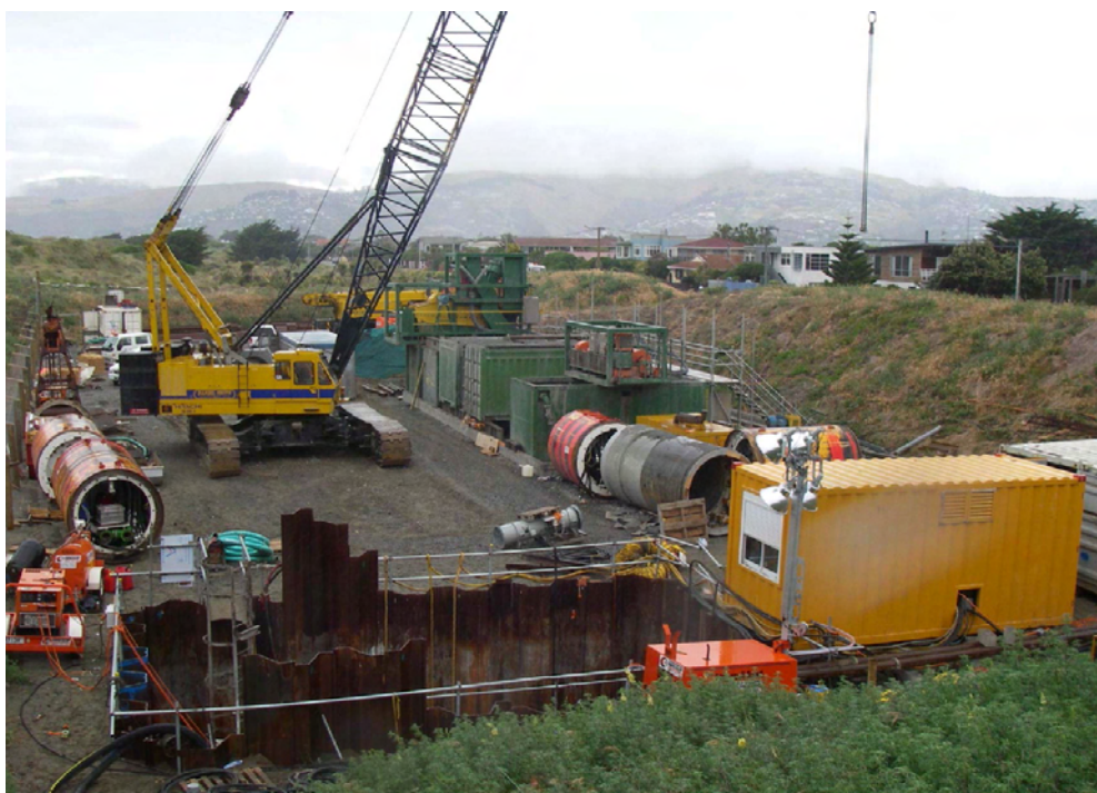
Figure 5 Typical microtunnel site (Christchurch)
