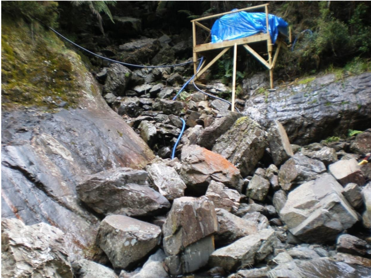
Figure 21. Water pump and bunded fuels above Sams Creek are covered to prevent rainwater filling bund.
