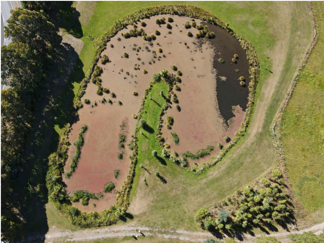
Figure 14. Constructed wetland at south end of proposed RERC alignment.
