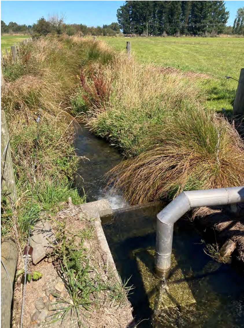
Figure 12. Middle Brook (looking downstream). An irrigation intake is located immediately upstream of a c.40 cm weir that likely prevents upstream and downstream fish passage.
