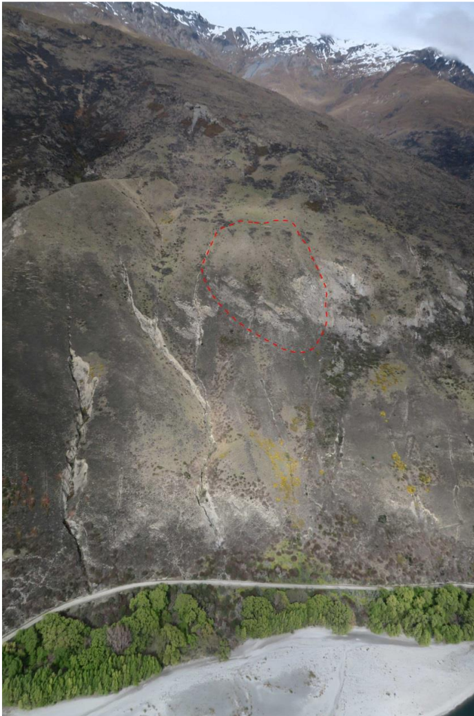
Oblique aerial view of the landslide area (red dashed line), looking south, with Chard Road and the Kawarau River bed in the foreground. (Photo: S Cox/GNS Science).
