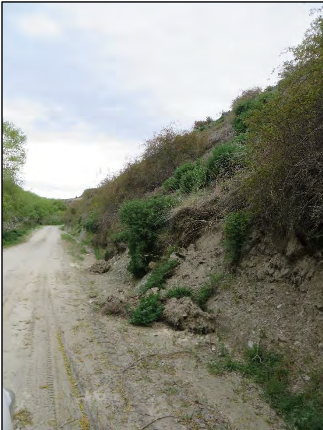
Photograph 9 (Left): Shallow landslide along access road (Chard Farm end of The Park)
