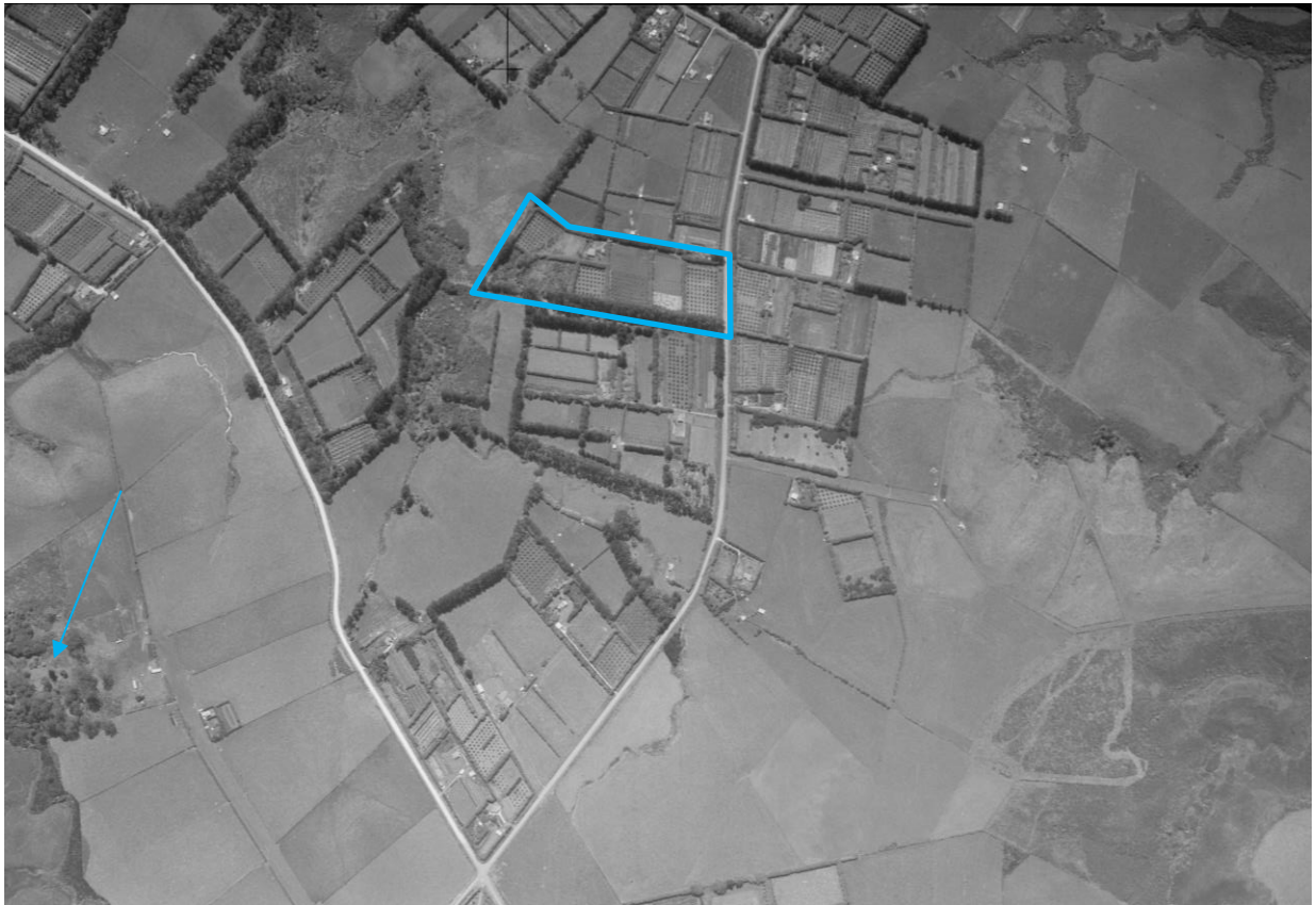
Figure 11: Detail from aerial image SN 209 Run 544/94 (1953) with well-established orchard on subject property (outlined blue), and Springbank homestead site (arrowed blue).
