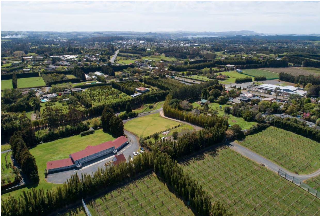
Plate 4. Kerikeri Park Lodge (red roofed building) and its relationship to the Site. The Site occupies mid-left of the image.
