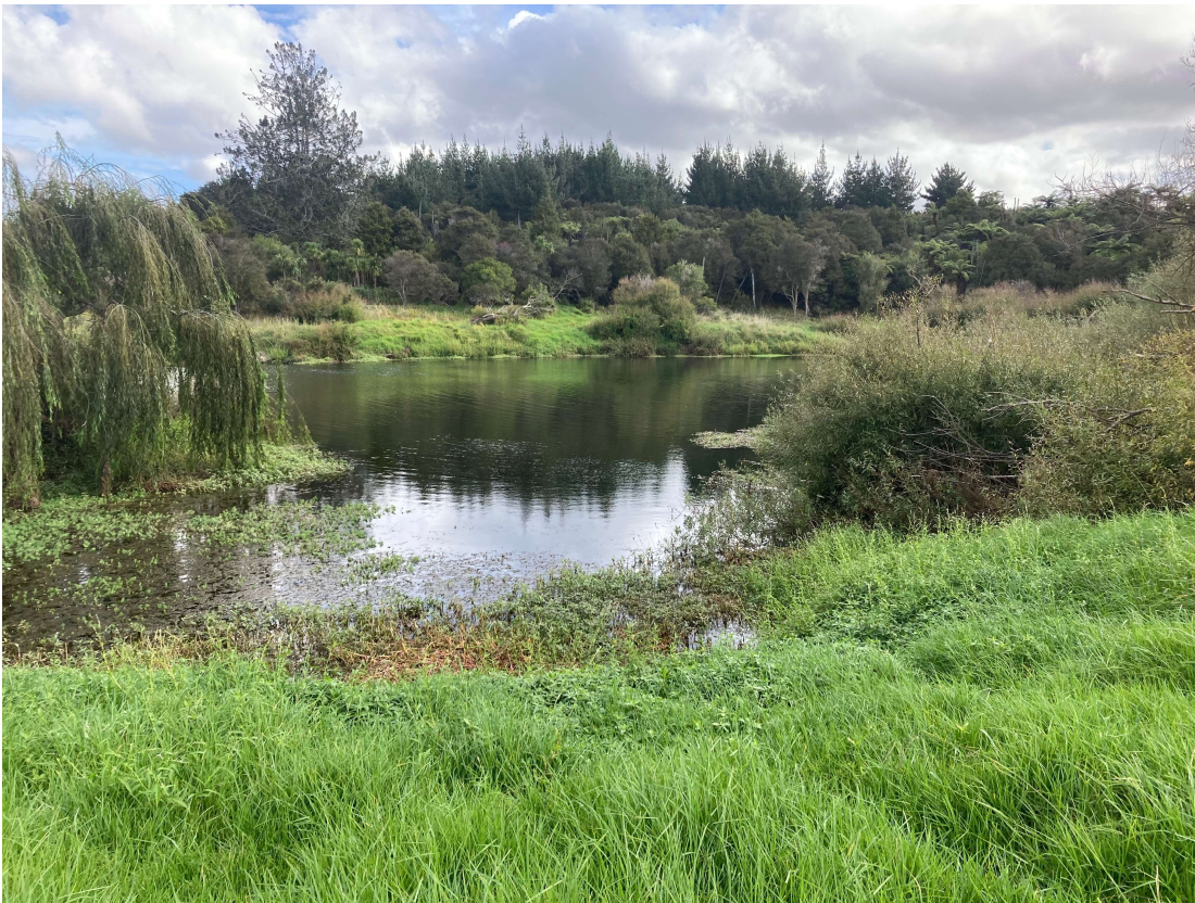
Figure 9: Around 100m downstream from the 9m deep scour hole below the falls, this scour hole forms a large pool. Screened, oxygenated water from the hydroelectric scheme would be discharged into this pool.
