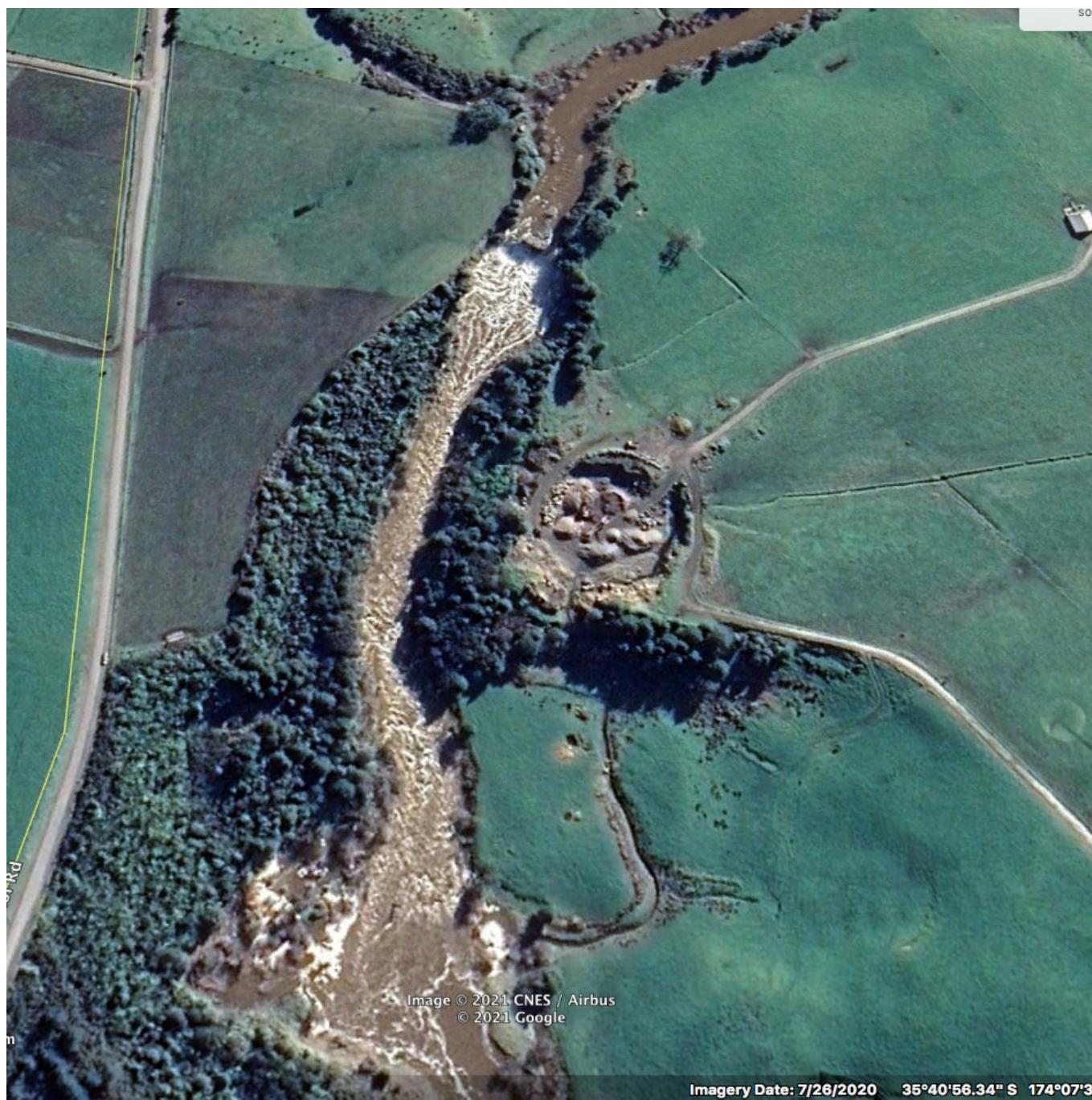
Figure 3: Showing the affected section of the Wairua River encompassed by the proposed Purua Falls hydroelectric scheme. On the eastern side of the river, the schemes water intake is around the top of the photo and the outlet back into the river is near the bottom of the photo. The river is shown in high flow following a substantial rainfall event.
