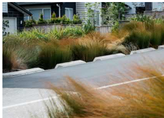
Stormwater management within streetscape
