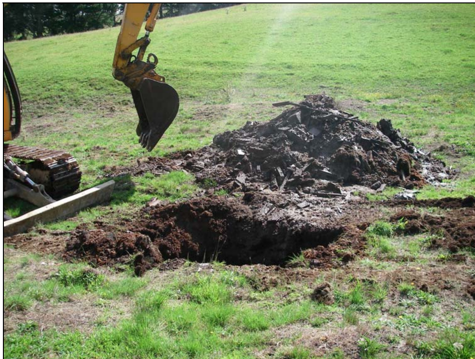
Plate 2: Typical Contents of Test Pits – Wood Fragments
