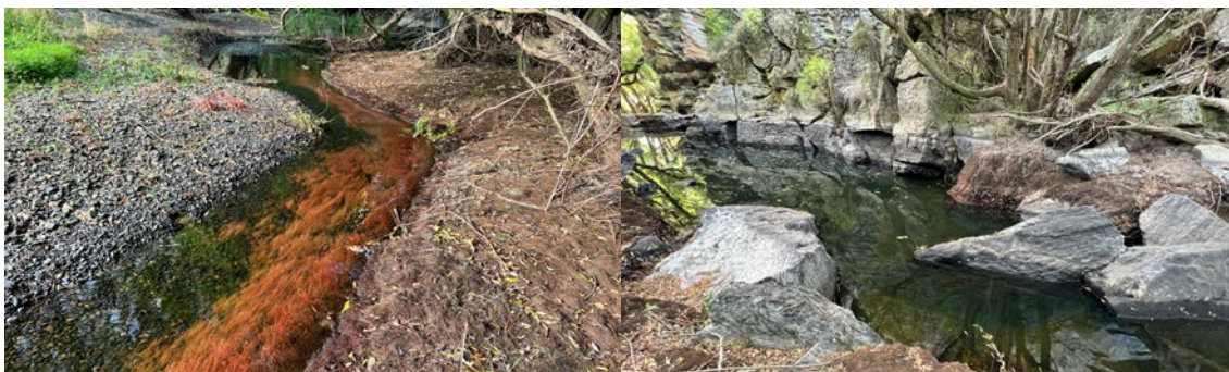
E. Extensive willow roots in the low flow channel.
