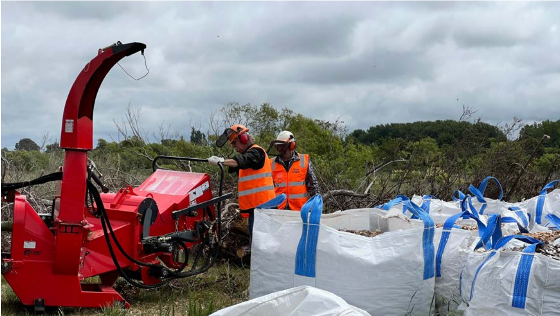
Figure 10 A wood chipper used by Mark Kruishoop to good effect in willow removal projects.
