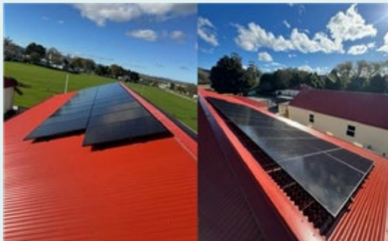
Turanga Waewae Pakura solar project.
