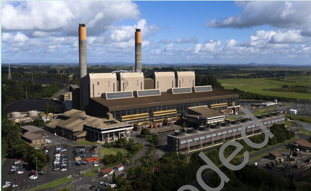
Image: Huntly Power Station
