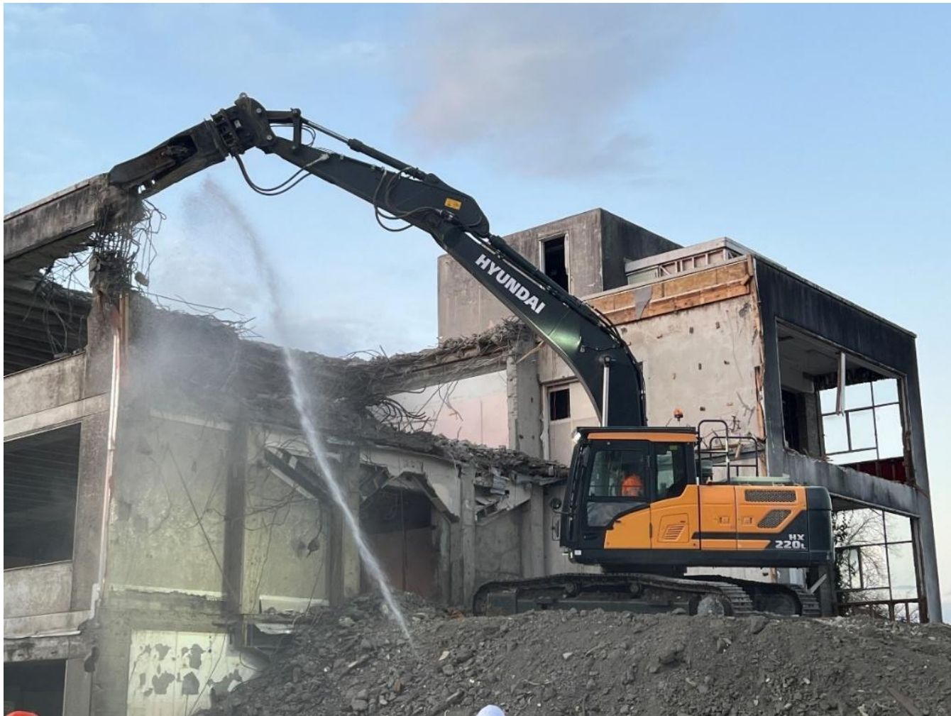
Photo: Demolition at Masterton Hospital. Source: Grün Group.
