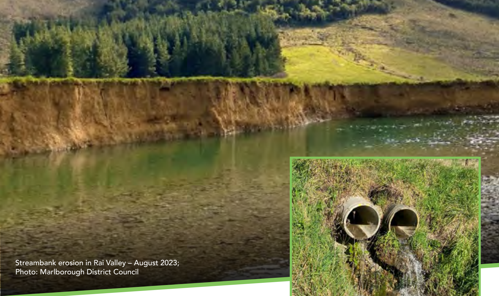
Culverts in Te Hoiere Catchment that are barriers to fish passage.
