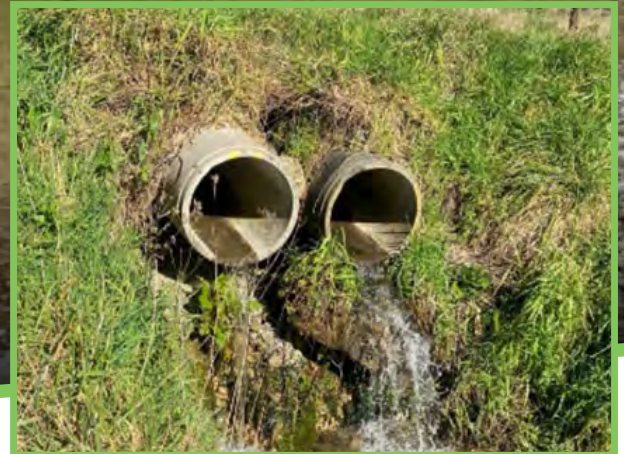
Culverts in Te Hoiere Catchment that are barriers to fish passage.
