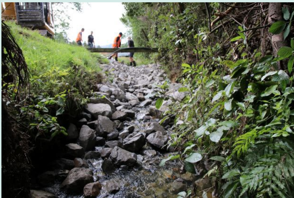
Image: Construction of a rock ramp fish pass in Shannon, Horowhenua
