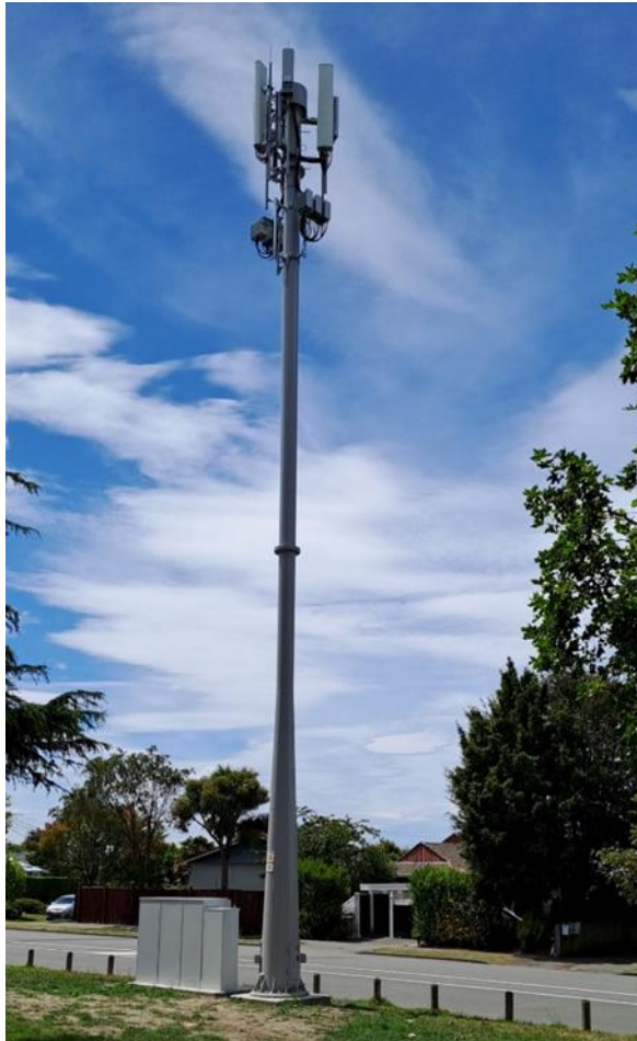
Figure 4: Example of a 1.6 m wide headframe on a 20 m pole in the road reserve in a residential zone in Christchurch (provided by Fortysouth)
