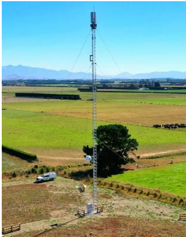
Figure 5: Example of a 35 m slim-line lattice tower outside of the road reserve in a rural zone (provided by the Rural Connectivity Group)
