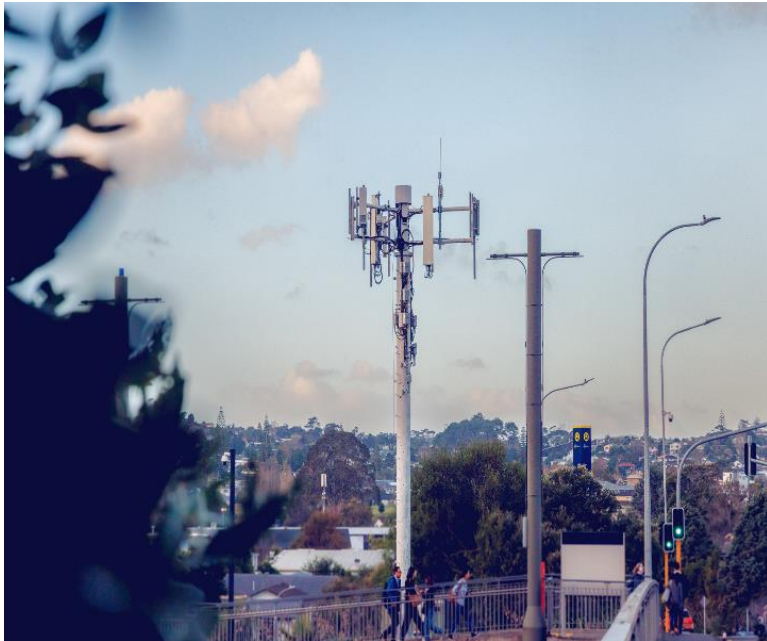
Figure 3: Example of a 4.5 m headframe on a 25 m pole outside of the road reserve in a commercial zone in Auckland (provided by Spark)
