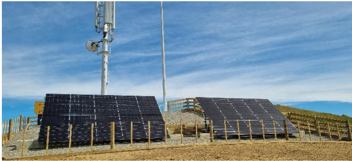
Figure 6: Solar panels on a Rural Connectivity Group site in a rural zone outside of road reserve (provided by the National Infrastructure Funding and Financing company)
