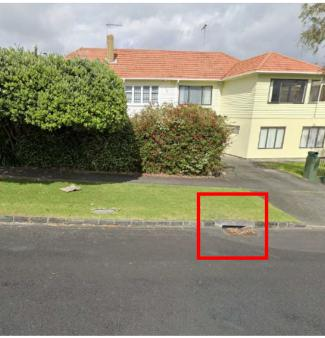
Proposed Stormwater Connection: New manhole to be installed where existing catchpit is currently located and drain the surface water flows for the site.
