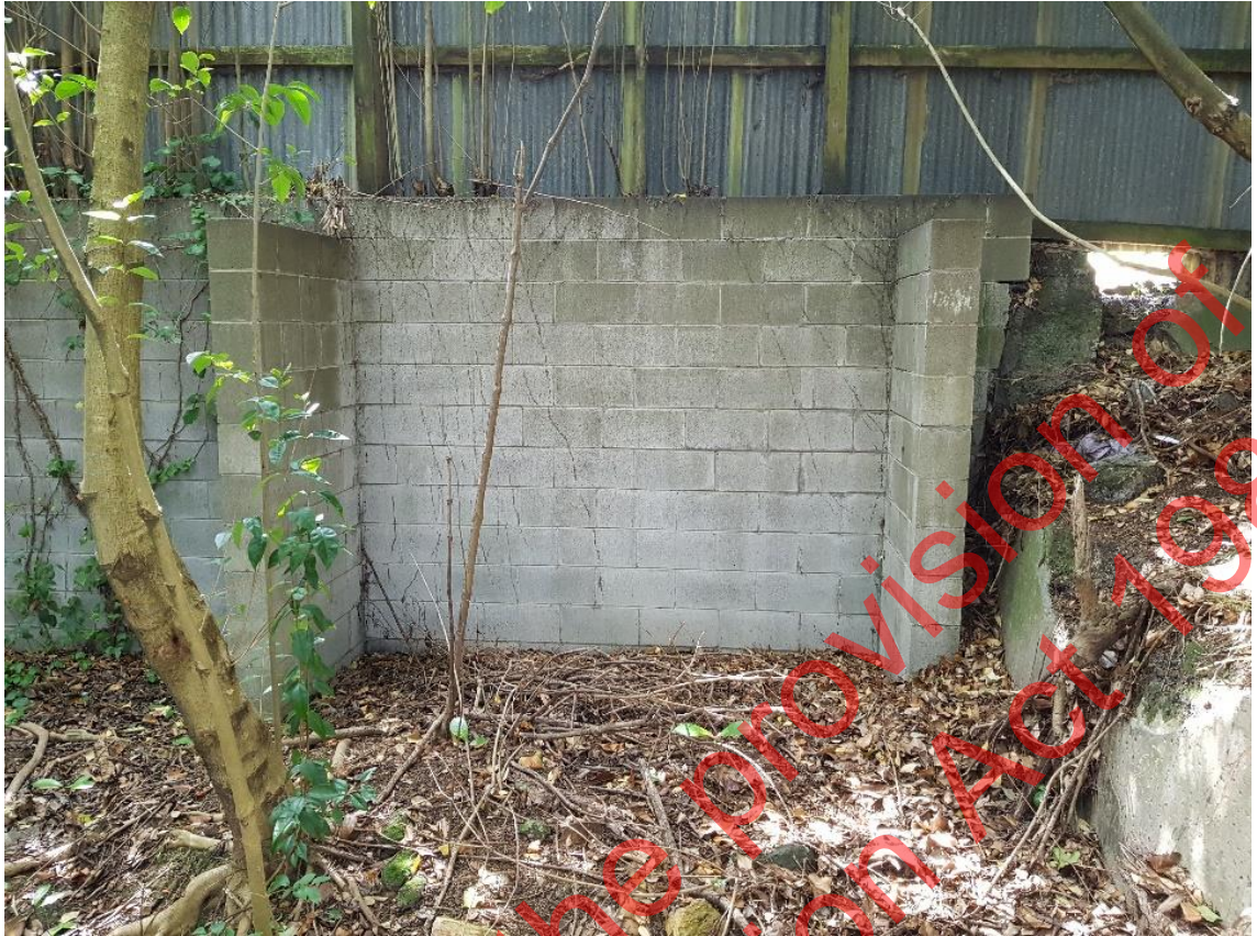
Figure 22. A retaining wall of concrete blocks adjacent to the feature is on the Ladies Mile boundary
