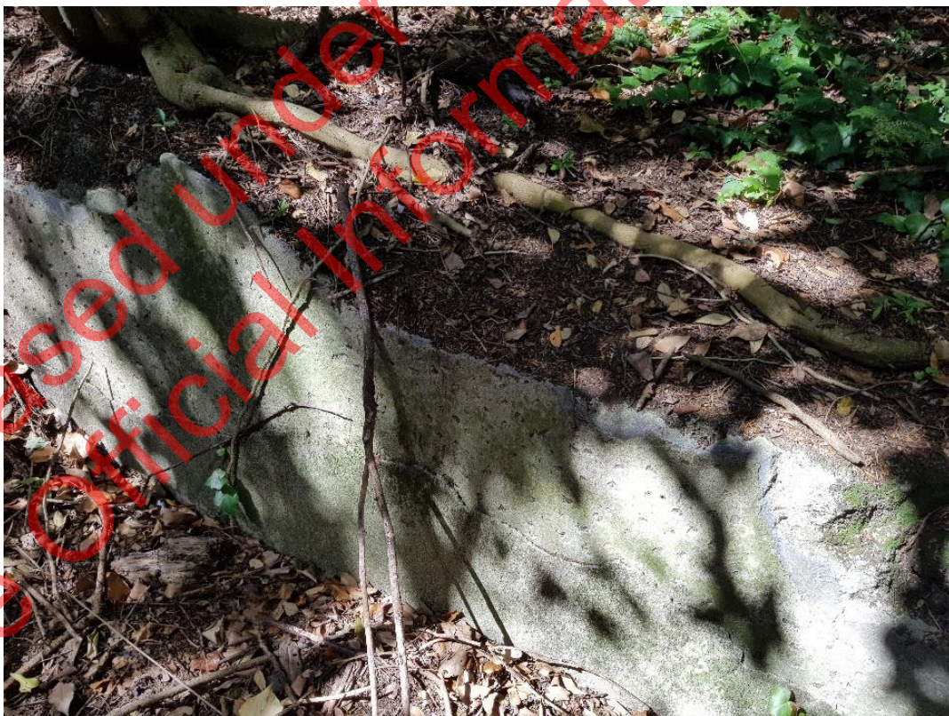
Figure 21. Close-up of one wall showing pecked surface (usually a preparation for plastering)
