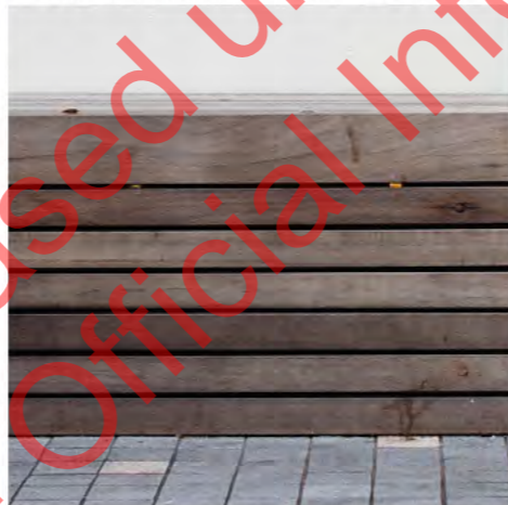
TIMBER SEATING 60 x 60mm Accoya battens on steel frame
