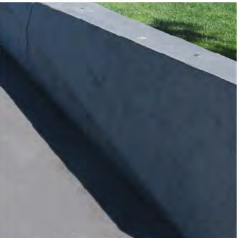
PRECAST CONCRETE WALLS/ STEPS/BLEECHERS Finish and mix to match Hurstmere Green; Nom. F5 precast concrete with colour additive. Lightly sandblasted and/ or honed finish.
