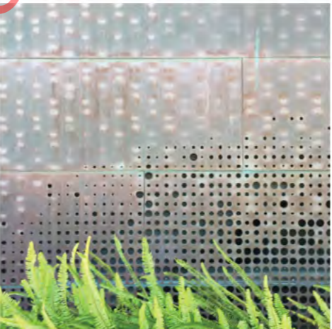
RAISED METAL CLAD PLANTERS 5mm powder coated aluminum panels fixed to concrete upstands/blockwork or 5mm powder coated aluminum freestanding planters supported on pedestals
