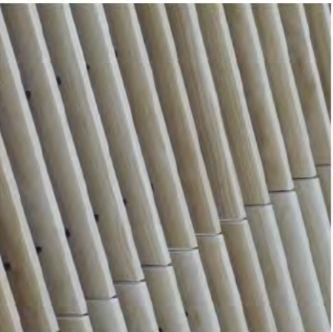
TIMBER BATTEN FENCING, GATES & SHELTERS 60 x 100mm Accoya battens with steel frame
