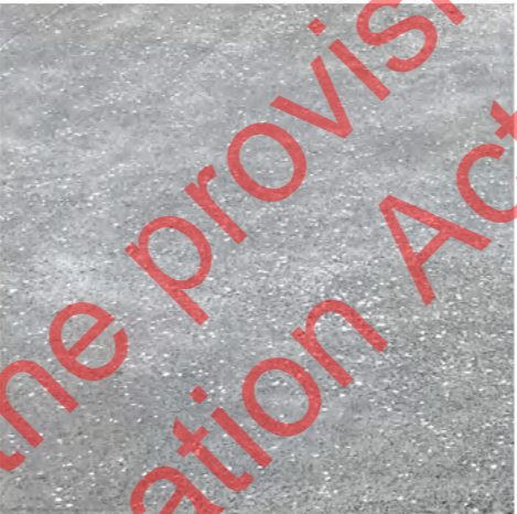
INSITU CONCRETE PARKING BAYS 150mm U5E insitu concrete 10mm basalt chip, lightly exposed aggregate finish, 4% Firth 'Haze' oxid
