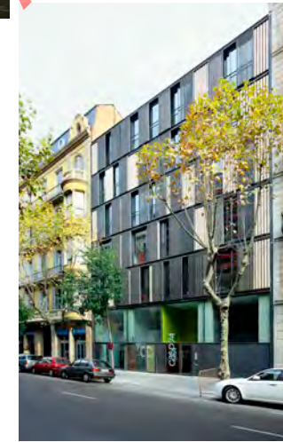
BARCELONA APARTMENTS, BARCELONA
