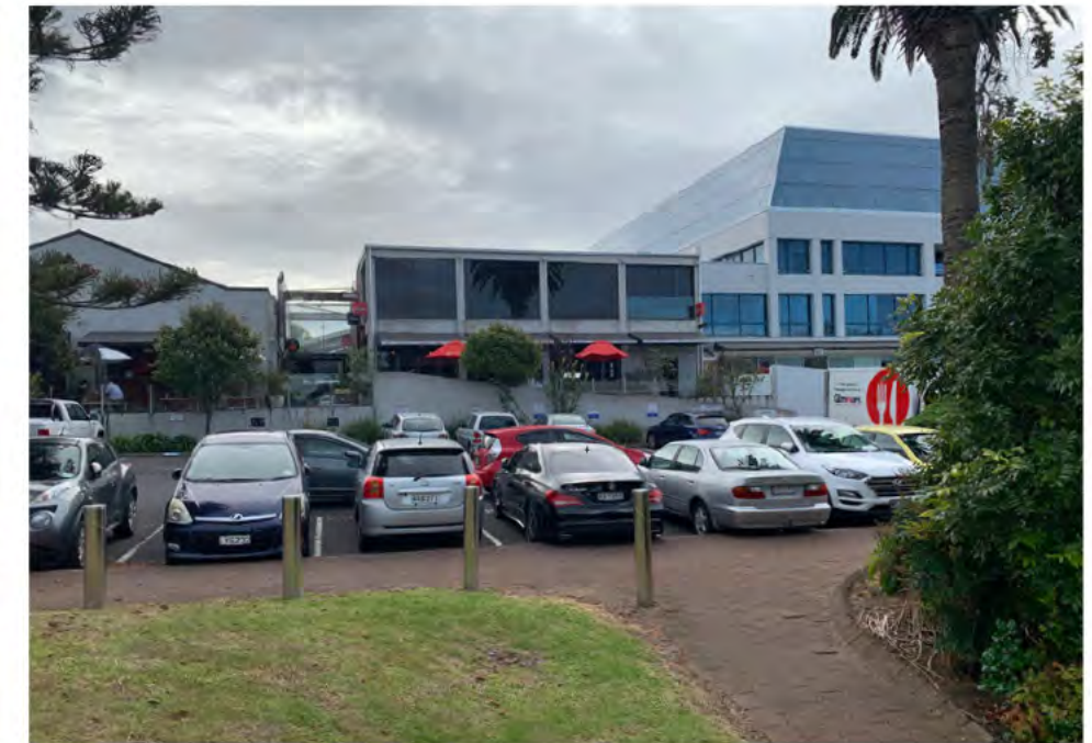
O / VIEW FROM CARPARK / TOWARDS THE WEST
