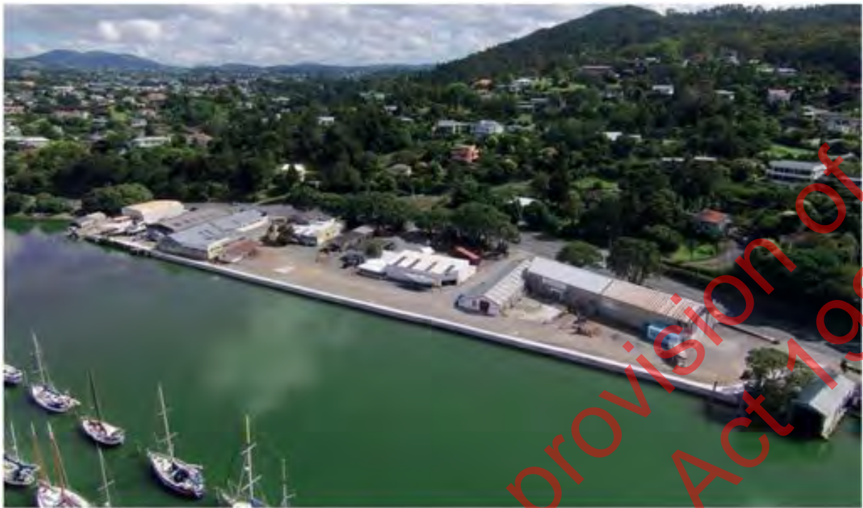
Figure 1: Existing Precinct site.
