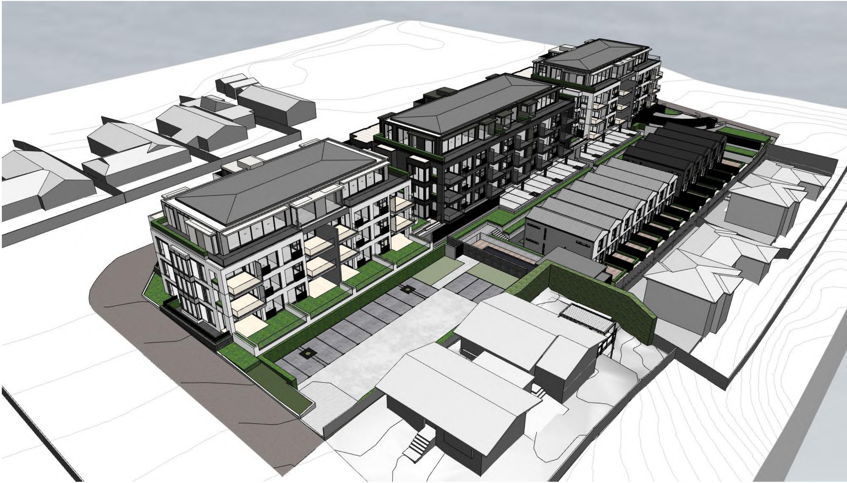
4 | AERIAL ( S E )
