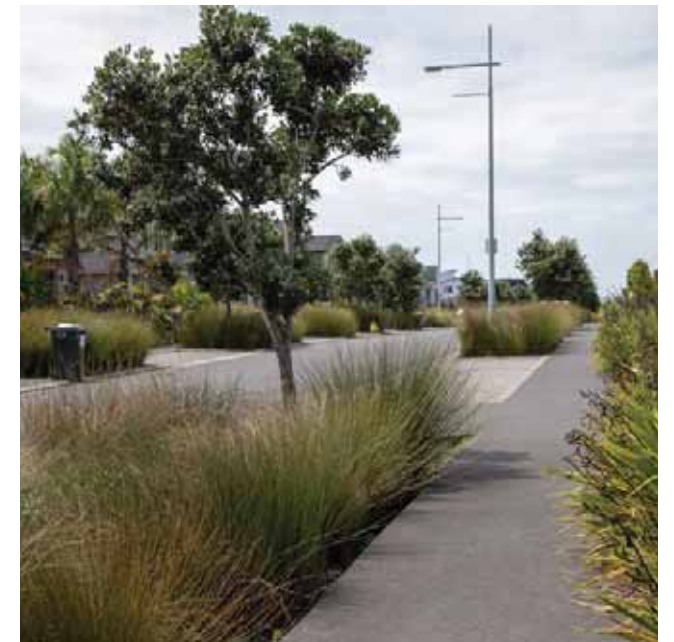
Stormwater treatment and planting along streetscape
