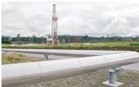
Figure 31 Geothermal drilling rig
