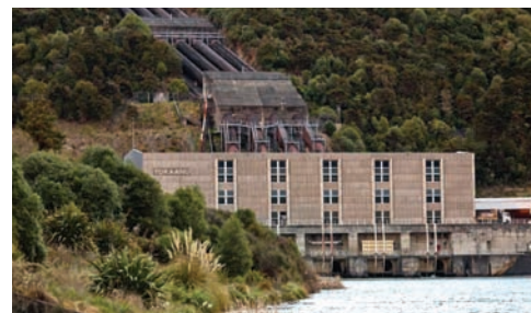
Figure 27 Tokaanu power station, Tongariro hydro-electricity scheme
