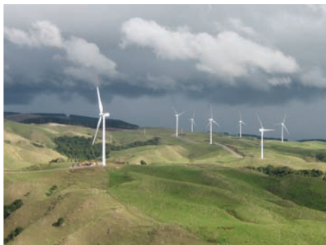
Figure 12 Tararua wind farm, Manawatu
