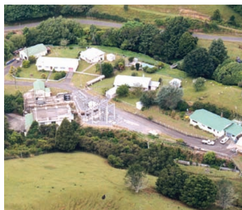
Figure 25 Motukawa hydro-electricity scheme, Taranaki
