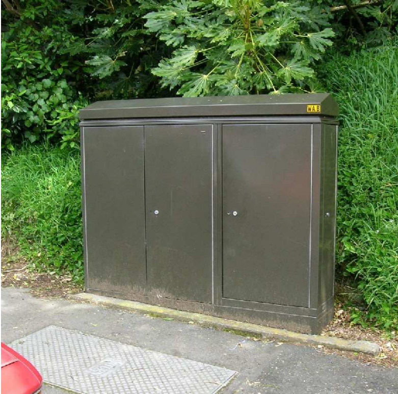
Typical roadside cabinet (Telstra – Saturn)
