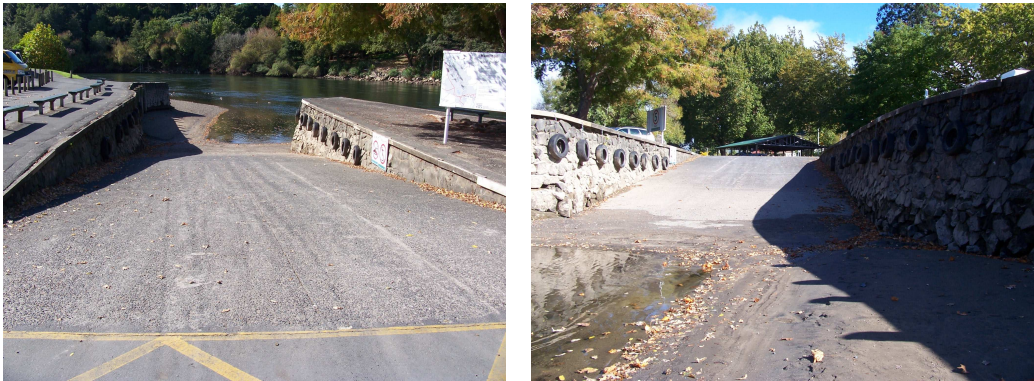
Figure 1: Roose Commence Boat Ramp (Hamilton) - BECA.
