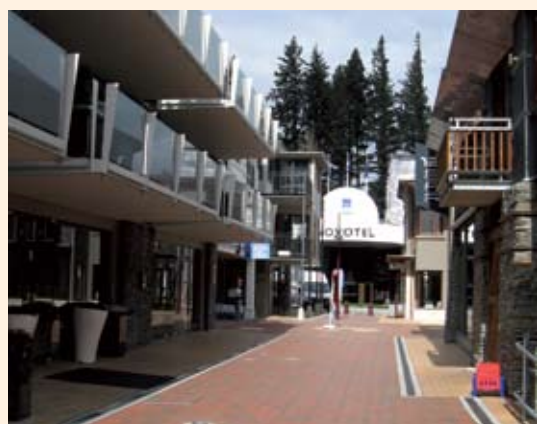
1 Looking into Church Lane between Williams Cottage (right) and Archer Cottage extension (left).
