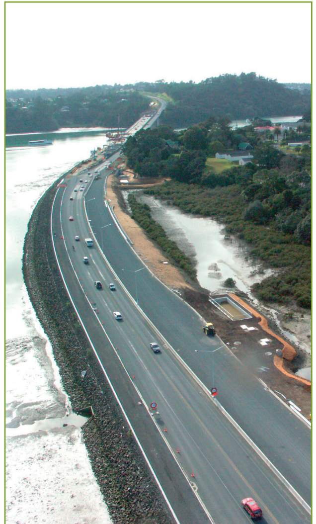
During the expansion of State Highway 18, it was raised an additional 0.3m to allow for predicted sea-level rise.
