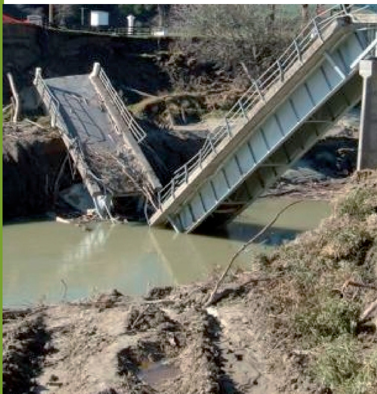
Mangamahu Bridge near Wanganui: Increased frequency of extreme weather events could lead to more cases of bridges collapsing.
