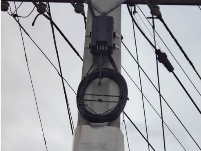
Figure A2.4: Photo showing fibre coil installation
