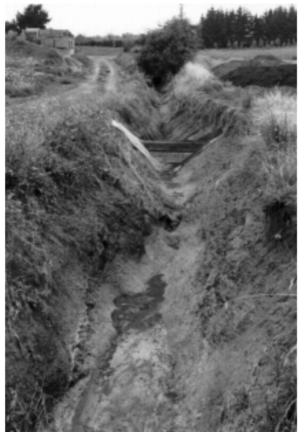
Photograph 9: Silt or sediment traps can be effective damage control devices where high amounts of sediment erosion can be expected. Cultivated areas, such as this vegetable growing property near Pukekohe, and forestry areas during harvesting are two situations where silt traps could be used. Silt traps must be regularly cleared of accumulated sediment to be effective.
