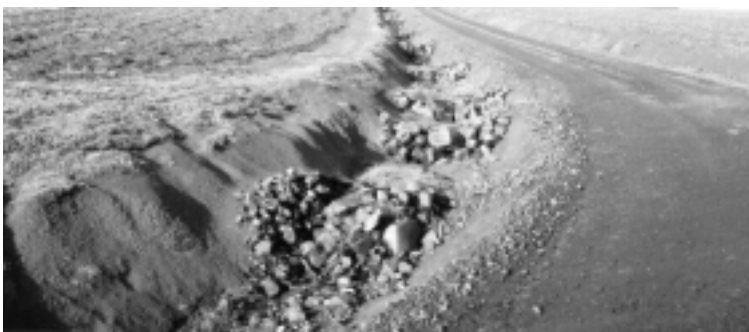
Photograph 58: Silt traps on AS Wilcox & Sons’ property near Mercer. Silt traps of this nature work well in trapping sediment and slowing down water flow, provided they are regularly maintained and emptied of accumulated soil.
