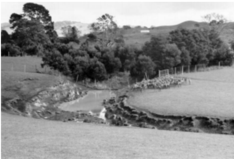
Photograph 33: This winter spring-fed depression has been cut out by deer and now generates a substantial sediment load each winter. On this Waikato property a wide (80–100 metre) grassy, permanently fenced riparian margin with thinned blackwoods above effectively traps most of the sediment, although in heavy rain the sediment load reaching the adjacent stream is significant.
