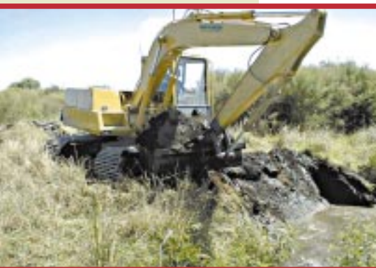
DIGGING THE SILT TRAPS
