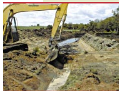
DIGGING THE NUTRIENT TRAP
