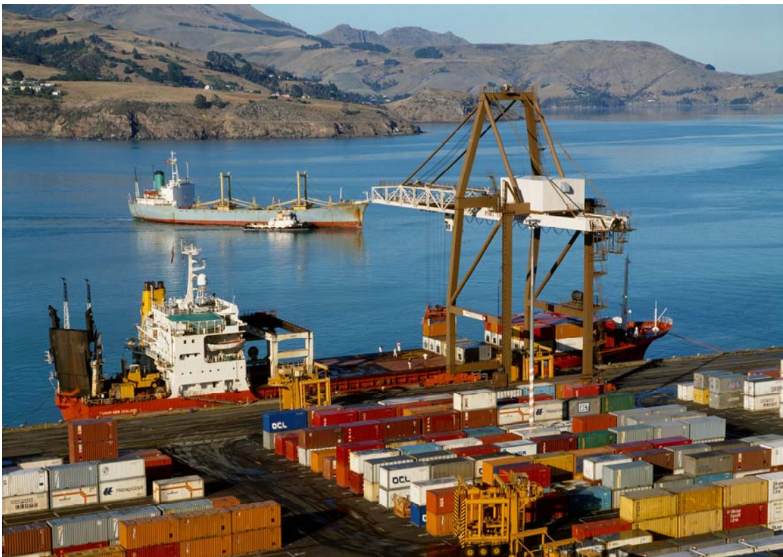
Container wharf, Lyttelton Harbour – PhotoNZ
