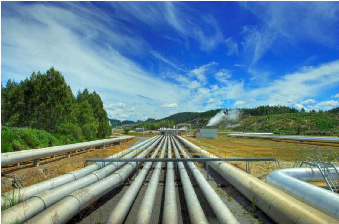
Wairakei Geothermal Power Station near Taupo – PhotoNZ
