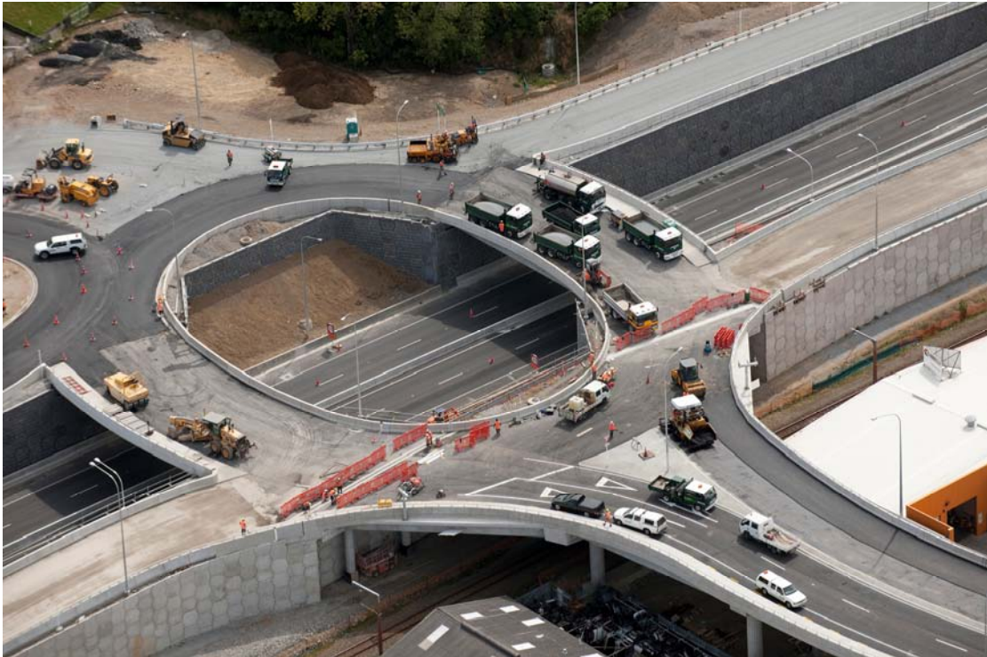
Dowse Interchange during construction, Hutt Valley – PhotoNZ
