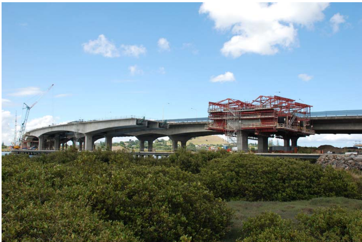
The new Mangere Bridge in construction, Auckland. Photo credit: Benjamin Paul AucklandMotorways.co.nz
