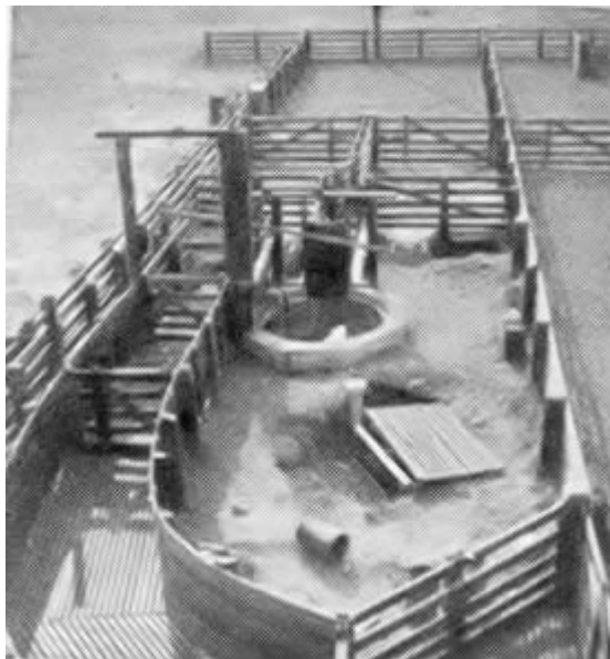
Figure A.6: Pot bath with curved race and covered sump
