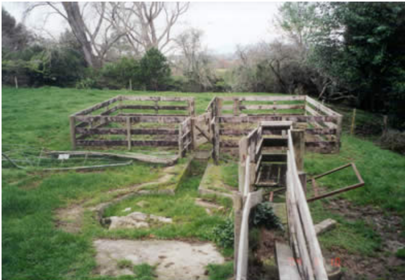
Figure A.9: Redundant pot dip with partially collapsed yards
