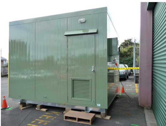
Figure 8: Example of a large telecommunication shelter able to be entered into by technicians
