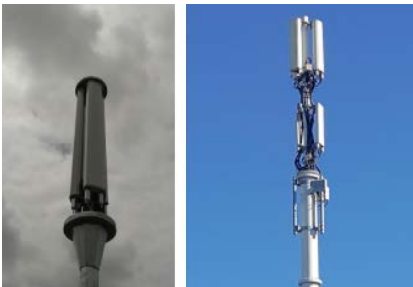
Figure 5: Examples of mounts used to attach non-dish antenna
