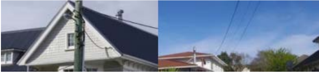
Figure 8: Aerial customer connection lines
