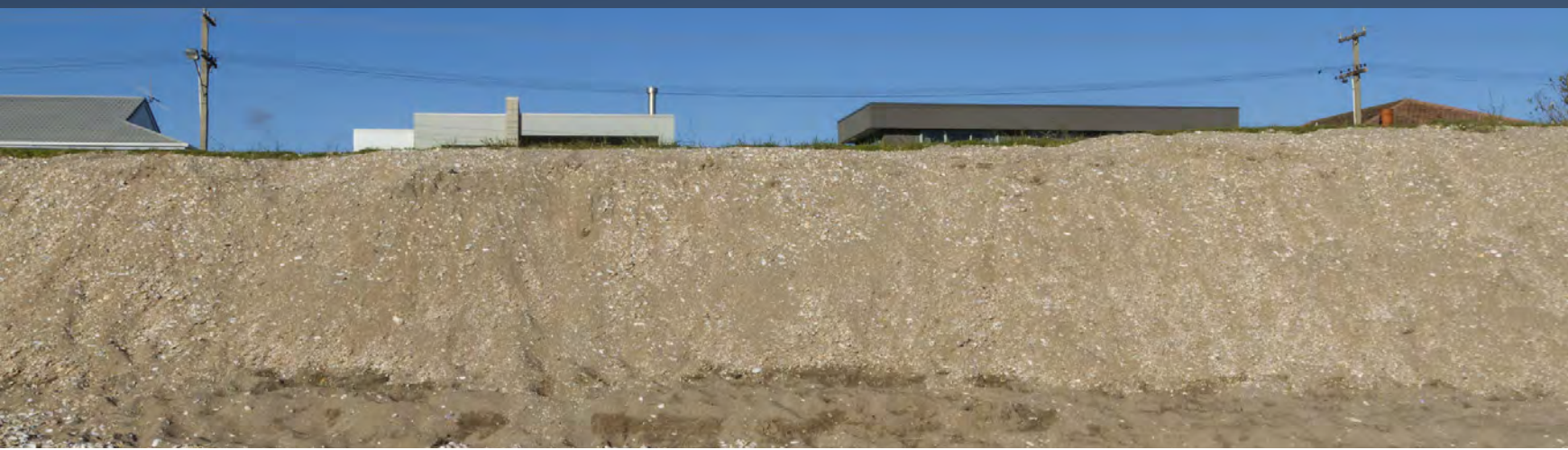
Dune erosion at Buffalo Beach, Whitianga
