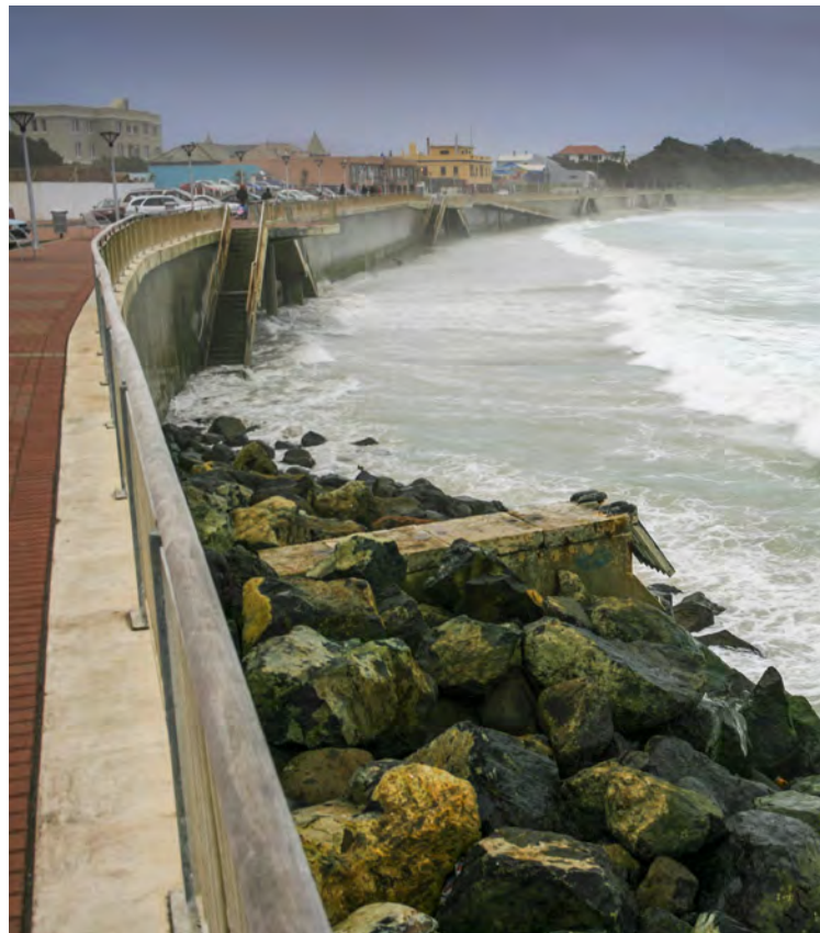
Seawall, St Clair Beach, South Dunedin
