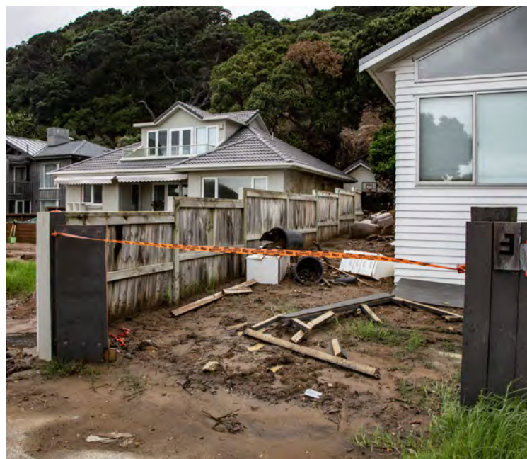
Slip-damaged houses at Piha
