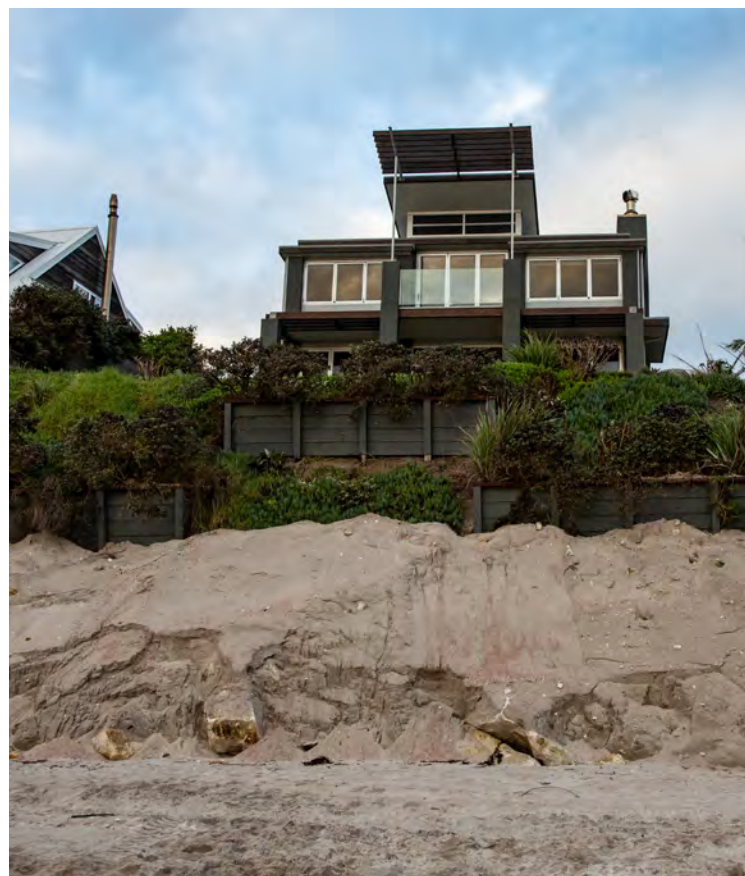
House subject to coastal erosion, Hahei
