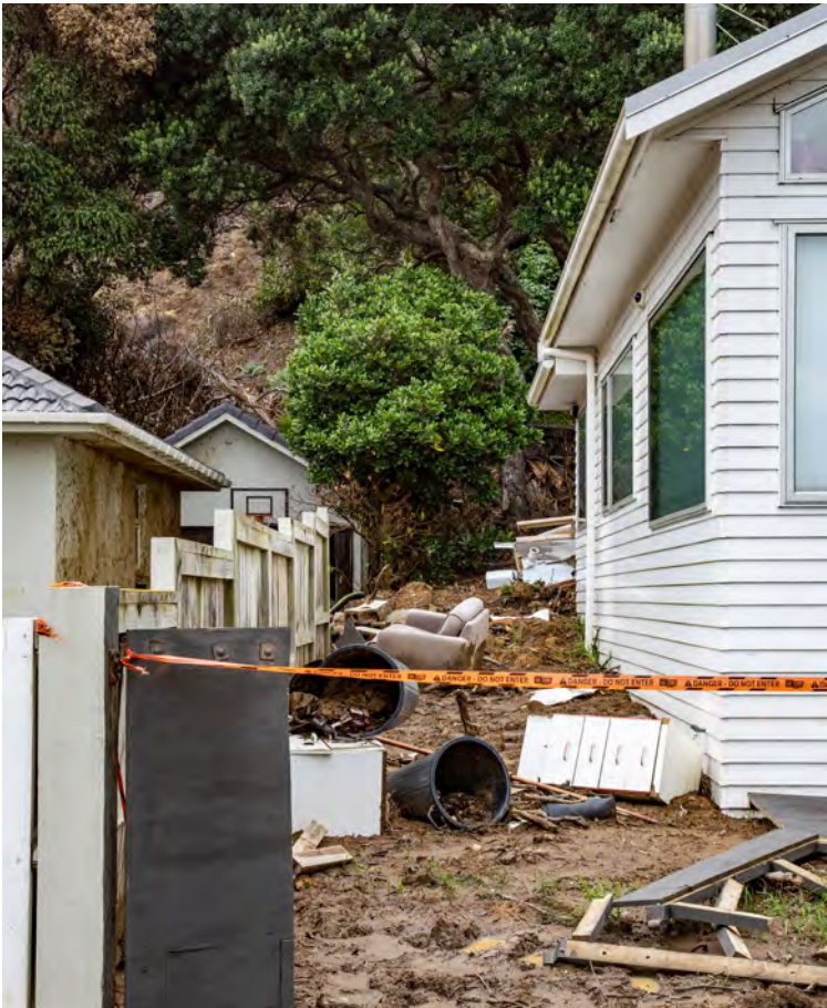
Slip damage, South Piha, Auckland
