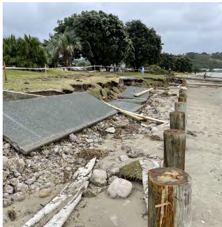
Coastal erosion damage to public walkway at Snells Beach (Neale Wills)
