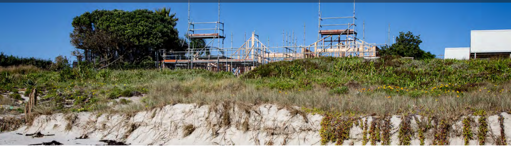
New build in hazard area, Matarangi
