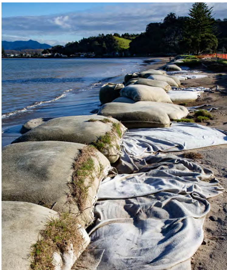
Erosion along Buffalo Beach, Whitianga
