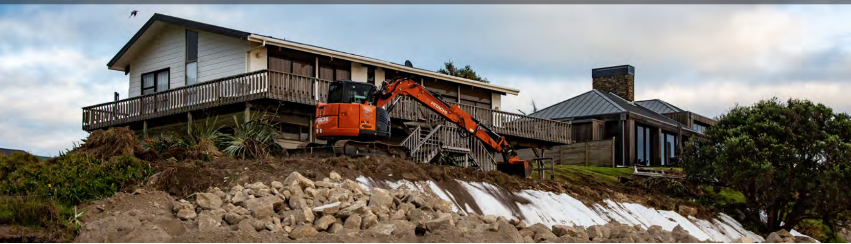
Coastal erosion impacting houses at Hahei
