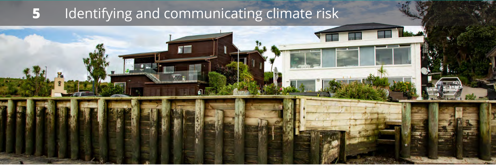
Clarks Beach seawall
