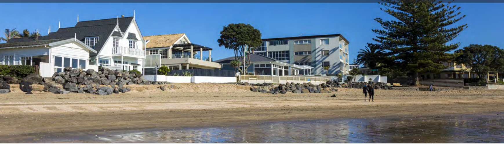
Various sea defences at Milford Beach, Auckland
