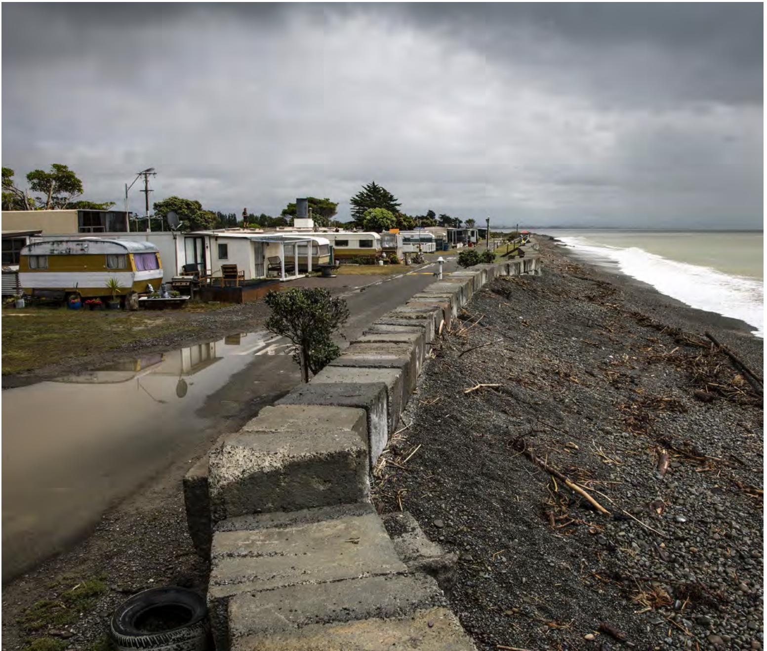
Coastal erosion at Clifton
