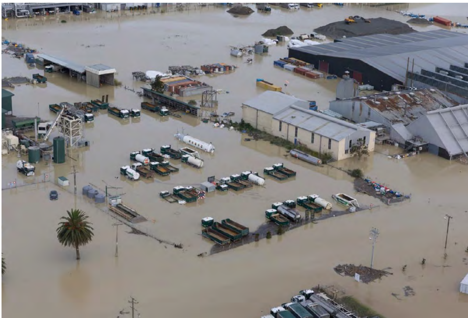
Flooded contractor's yard, Hawkes Bay (Waka Kotahi)
