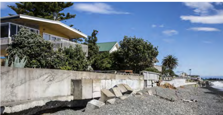
Coastal erosion, Haumoana
