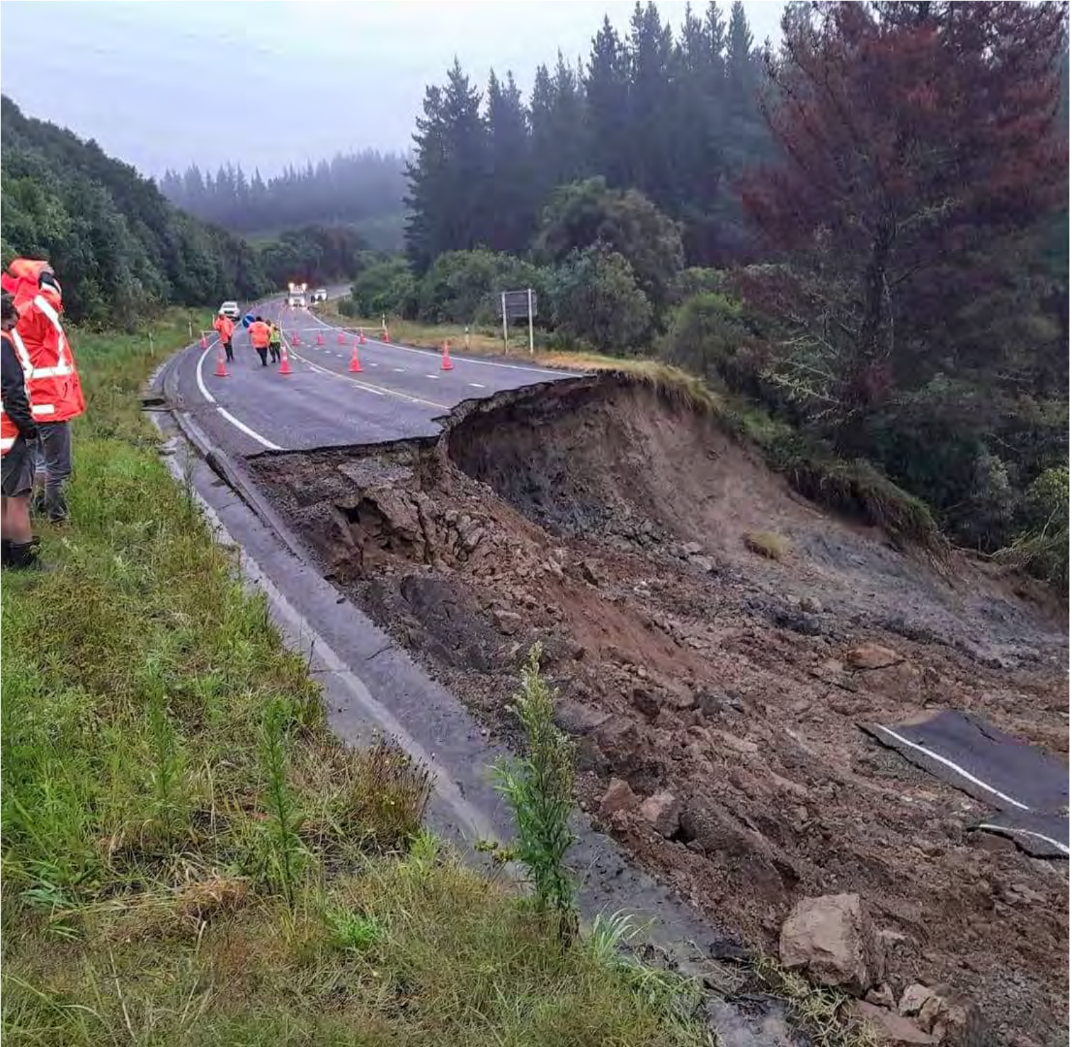
Collapse of State Highway 5 due to flooding, Hawkes Bay (Waka Kotahi)
