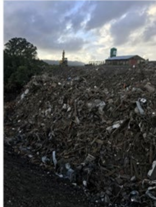
Before: Facing North, Looking at Tip Off Area
