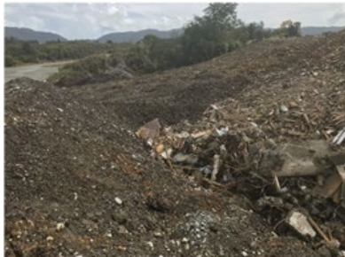
After Saturday covering, Facing West
