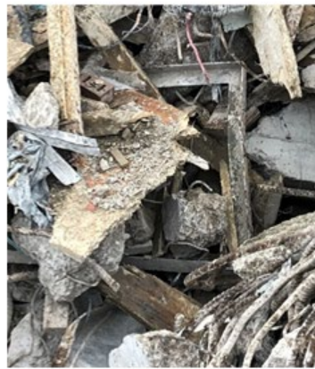
Exposed Metal Framing
