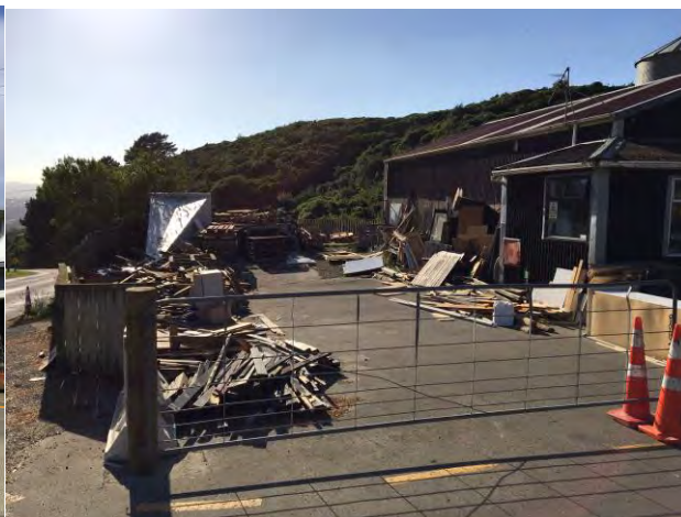
Figure 3.4 Existing public C&D building
