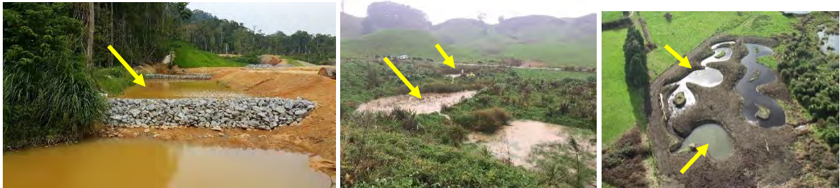
Figure 4-6: A range of sedimentation traps with differing degrees of landscape fit. Sedimentation traps can be built solely with functionality in mind (left), or integrated with wetlands (two examples on right). The sedimentation traps are arrowed.
