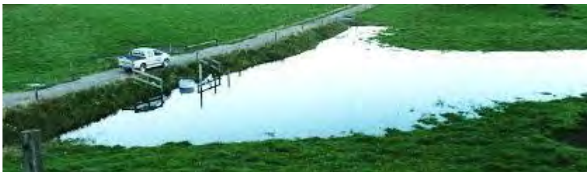
Figure 4-8: Pondered drainage temporarily impounded behind a detainment bund created from a causeway road. From Clarke et al. (2013).
