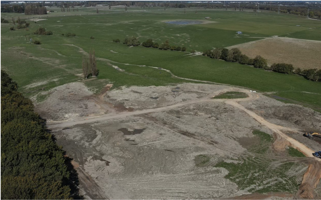
Chesterhope Station – Franklin Road (05-04-2023) and (05-05-23)
