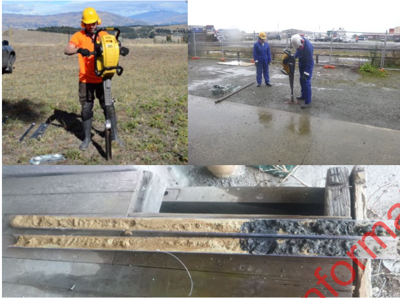
Figure 7: Window Sampling Equipment and Cores
