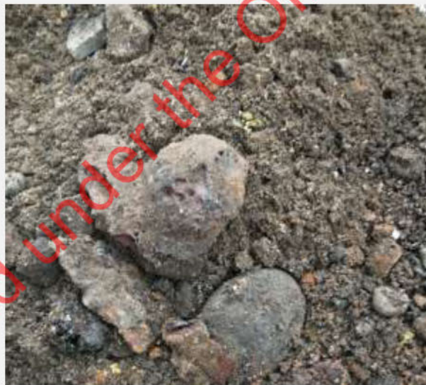
Image 3 – Foundry slag within fill material
