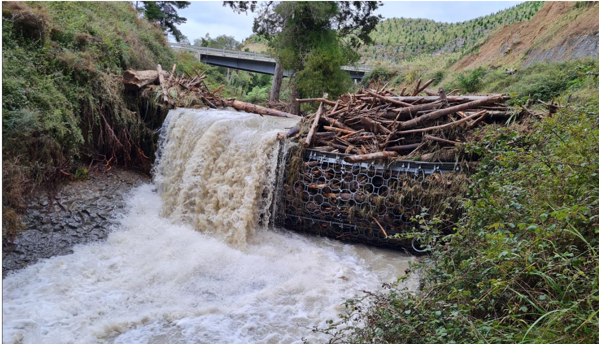
photo courtesy of Matariki Forests Ltd, Hawkes Bay – Consented ‘net type’ slash trap
